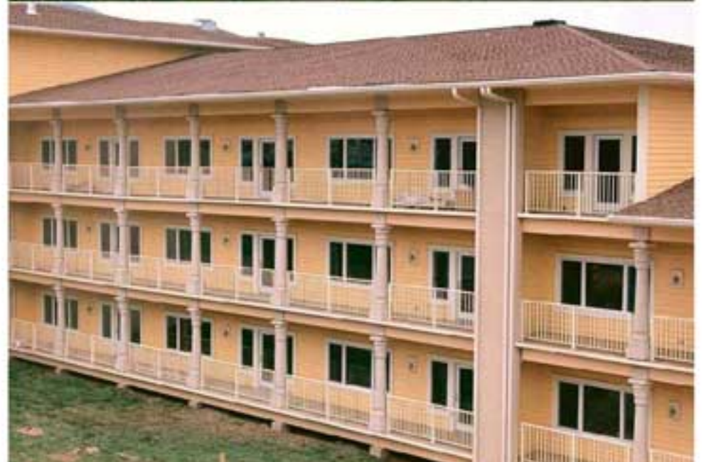
Main Building, Detail
